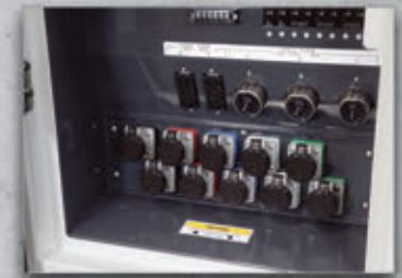
2 | Single-Phase Receptacles 120V - 20A x 2 | 240V - 50A x 3 Optional Dual Row Cam-Loks™ Shown
